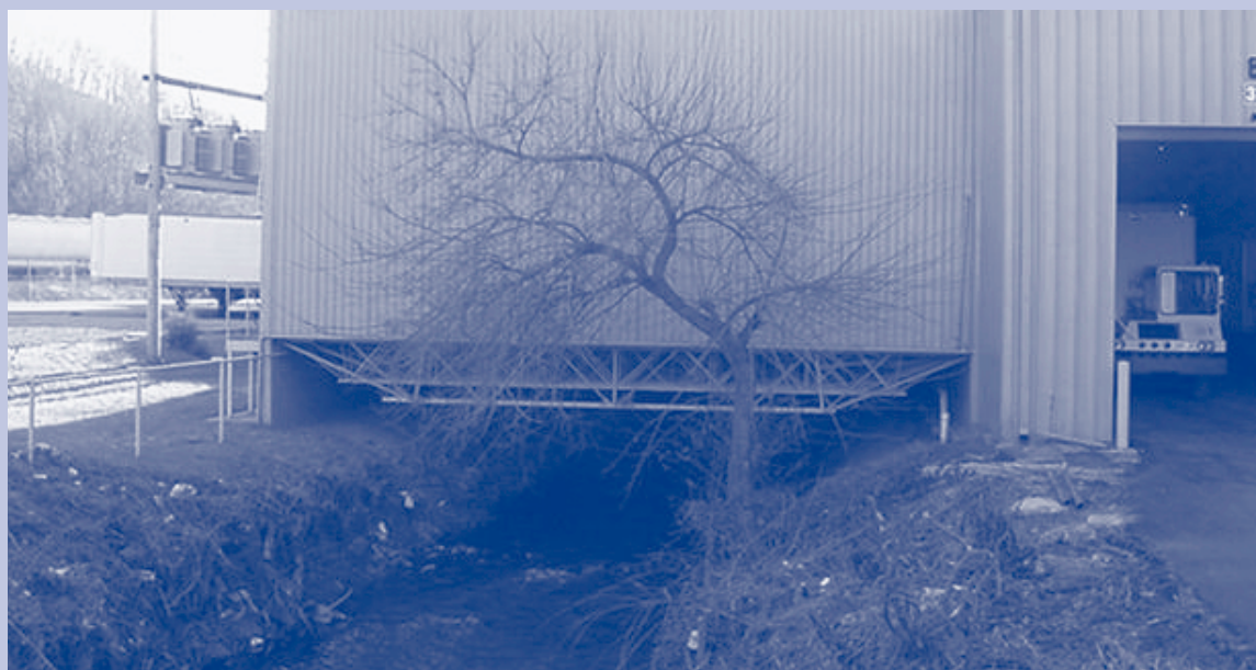
Creek that Supplies Cool Intake Air to Compressors
