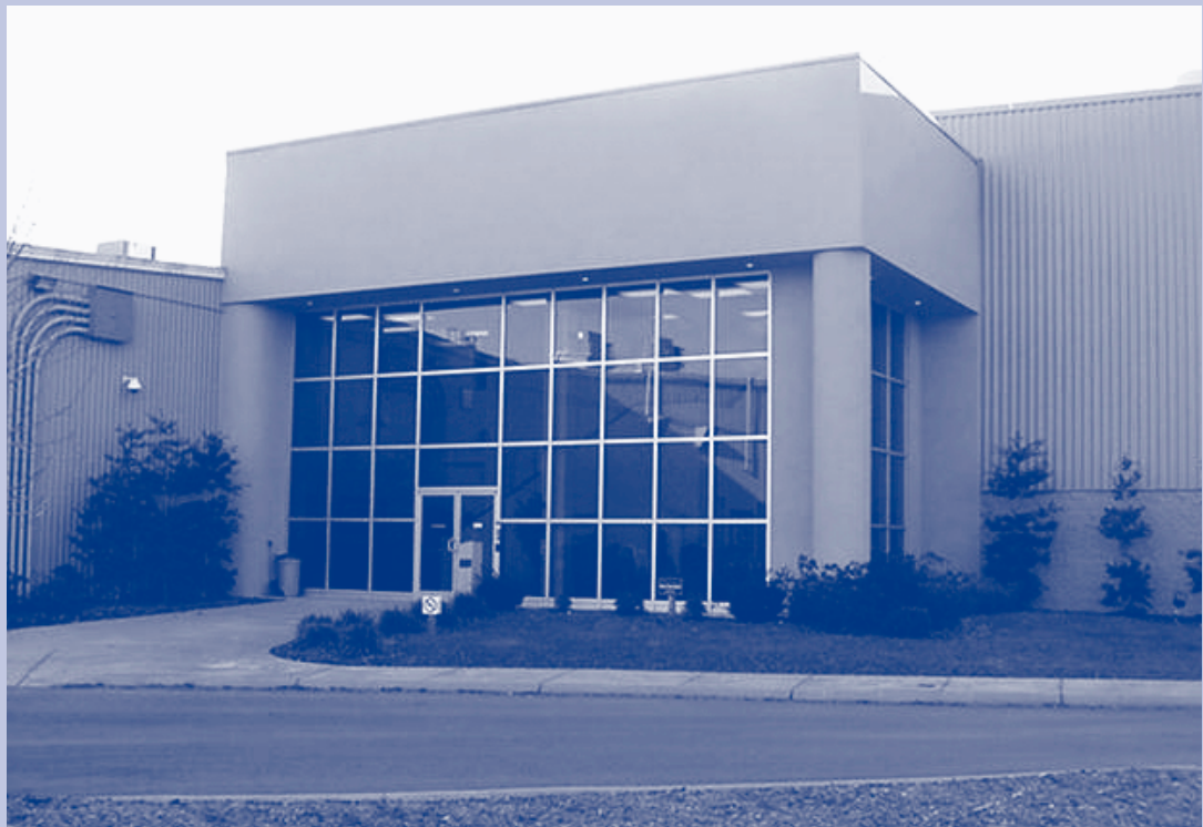
Front Entrance to American Water Heater Plant
